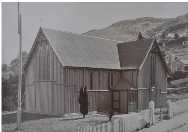
St Saviour, West Lyttelton, 1940, from the south-east.
